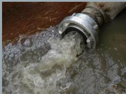
■ Step 3: Start pumping
