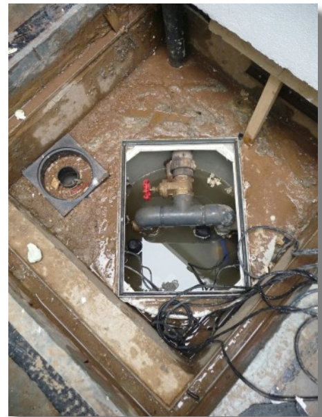
Pumpmatic Packaged Pump Station
