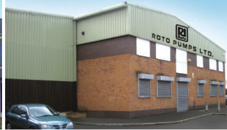
Manchester Office & Warehouse
