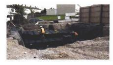
regular inspection and maintenance of the soakaways and comply with local authority highways and drainage guidance with a view to adoption by the council. Stormbloc® Inspect's inspection chambers and access tunnels in the soakaways are fully integrated within the modular block system to ensure simple installation and connection to the surface water drainage system, as well as easy access for ongoing maintenance.
