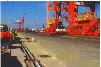
578 metres of Hauraton FASERFIX® SUPER 150, channels have been installed along the redeveloped quayside and container handling area at the Royal Portbury Dock, Port of Bristol.
