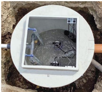
effluent, single and twin, below ground pumping station, the FE-Matic. This is available as bare tank or assembled with single or multiple pumps.
