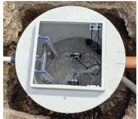
effluent, single and twin, below ground pumping station, the FE-Matic. This is available as bare tank or assembled with single or multiple pumps.
